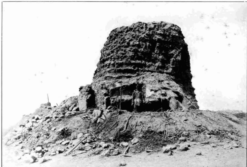
180. ANCIENT WATCH-TOWER T. XIII, WITH QUARTERS, TUN-HUANG LIMES, SEEN FROM SOUTH-EAST, AFTER EXCAVATION.
